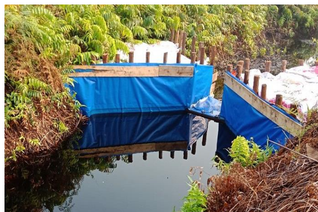
Figure 2. The construction of drainage canals at the research site that has been built by Astiani et al. (2020)
